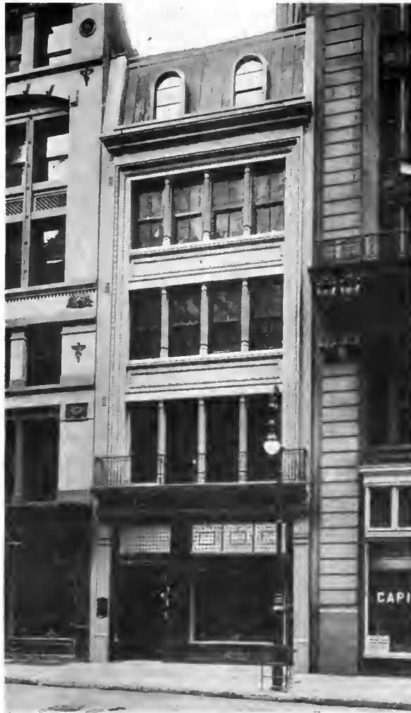
EXTERIOR OF BUILDING AFTER REMODELING
